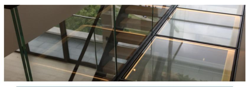
Manufactured using chemical etching, anti-slip floor glass provides solutions to incorporate the design flexibilities of glass with the functionality of traditional flooring materials. Implemented via special combinations of raised and recessed areas, the surface also maintains a high level of anti-abrasion resistance ensuring suitability to high-traffic applications whilst safeguarding the longevity of the product.
